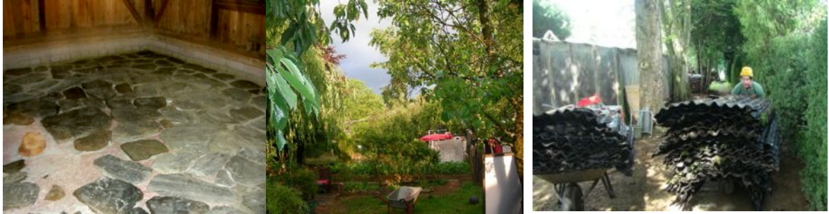
slades, spinach & radish and roof-removal.....
